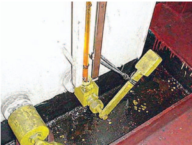
Self-closing gauge glass held open with string
